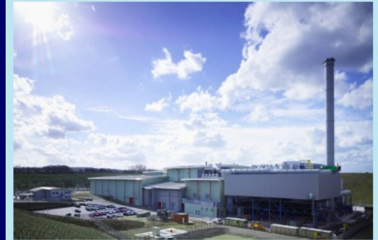
Allington Energy from Waste (EfW)
